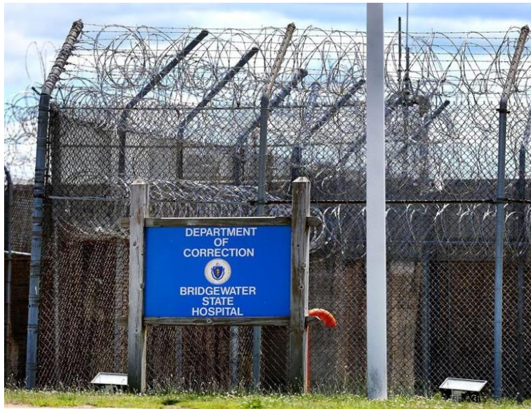
Exterior barbed wire fence and exterior sign at Bridgewater State Hospital.
